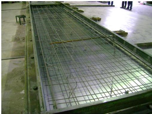
**Figure 12: Lightweight SCC is often used for large wall panels.**
