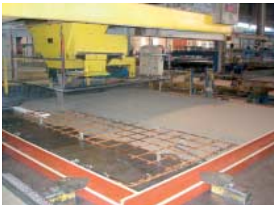
Fig. 5 Light-weight SCC is often used for large wall panels.
