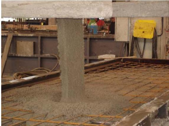
Figure 6: Casting of the L-SCC.
