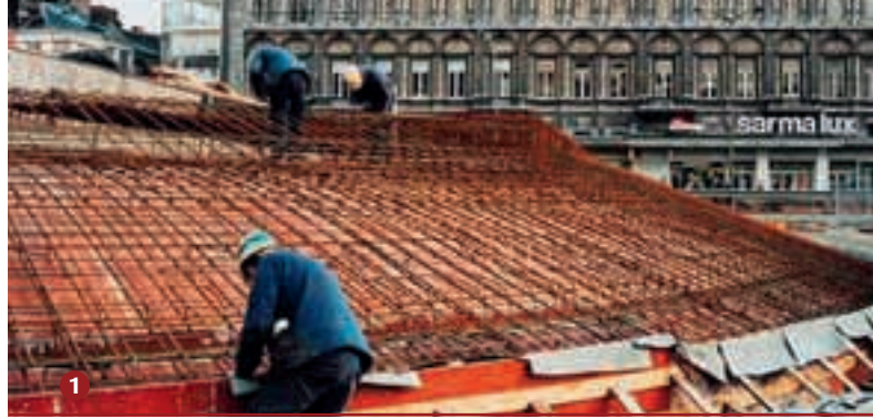
Archeoforum in structureel lichtbeton (Place St-Lambert - Luik)
