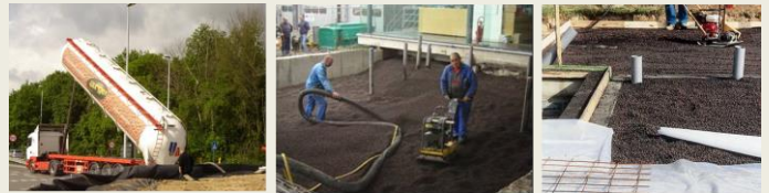
Figure 3: Blowing with vibrating plate levelling-compaction installation
