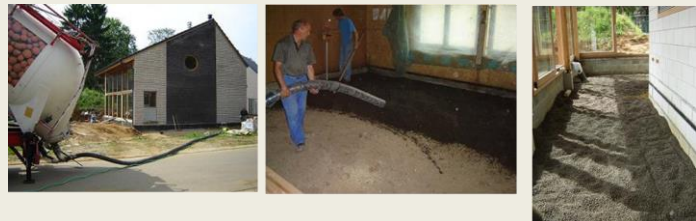
Figure 4: Blowing with manual levelling installation
